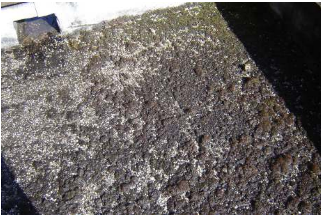
Flat roofs on the east side of the building.
