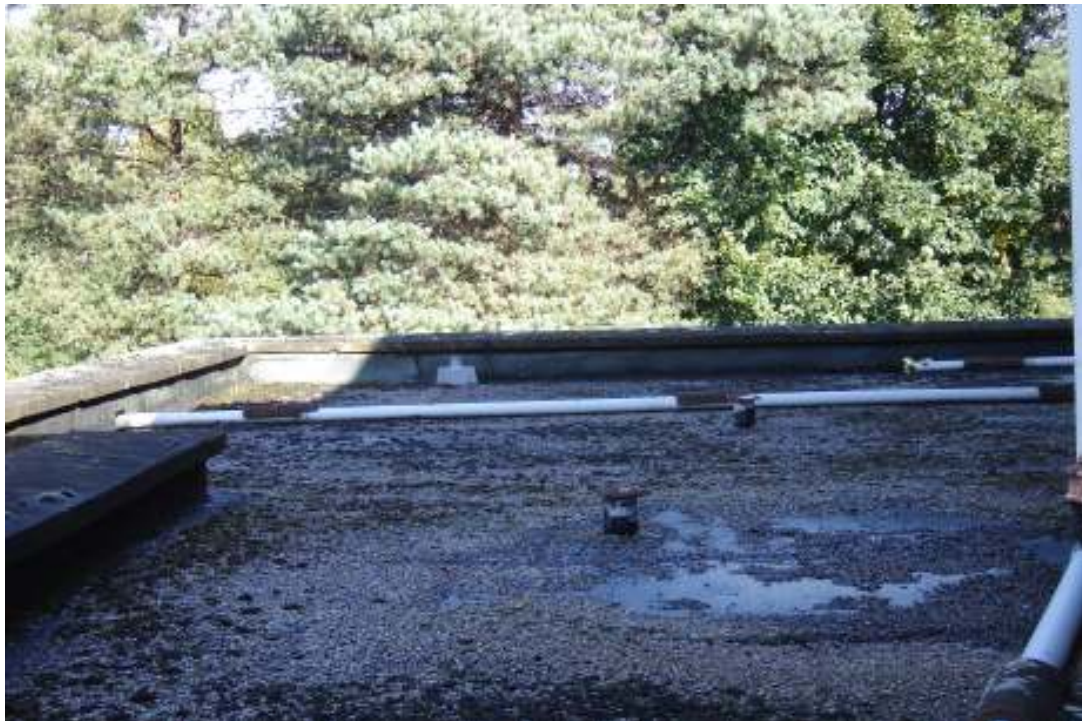
Flat roofs on the west side of the building.
