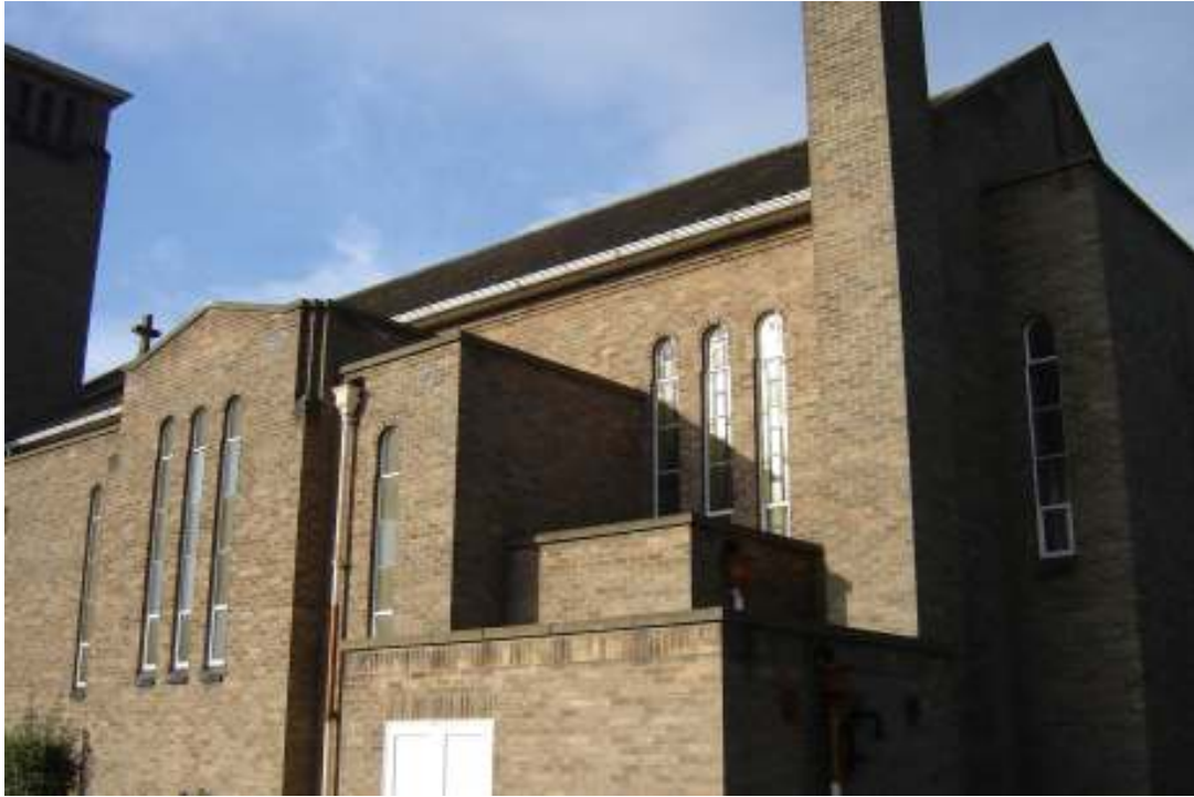
Areas of flat roof north east corner.
