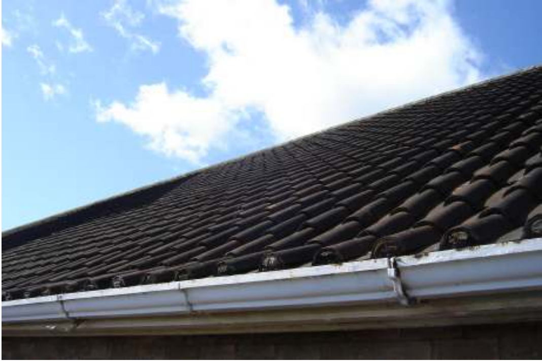
Main roof of church photographed from the East.
