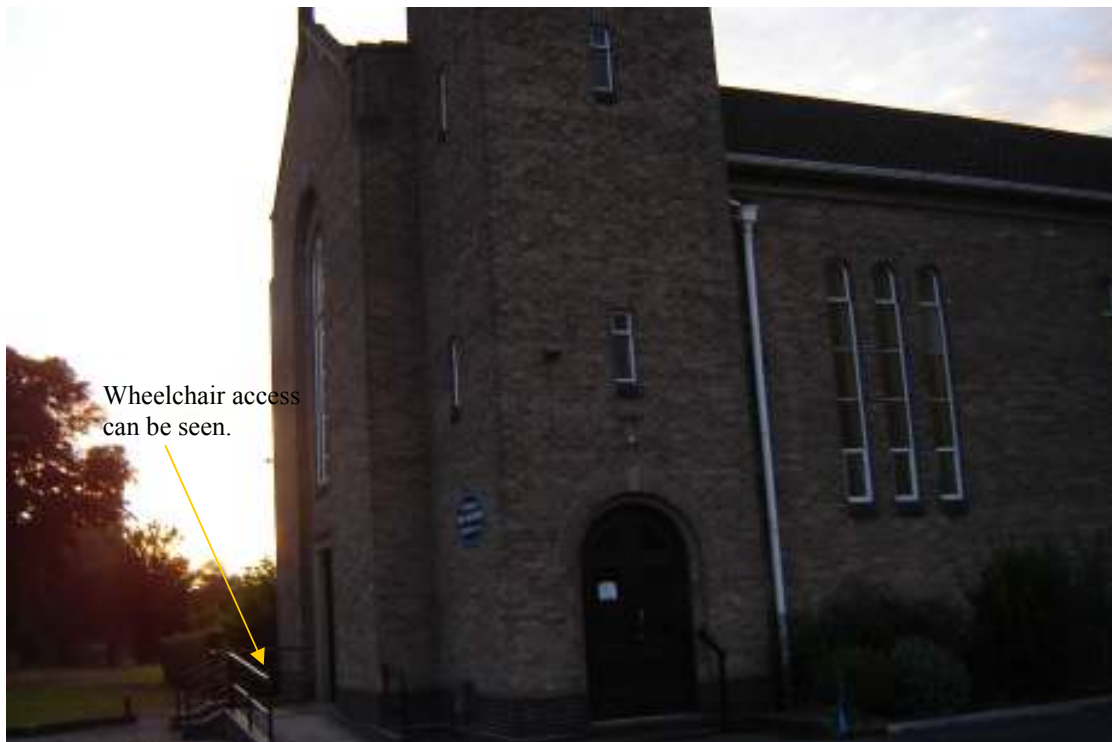
South east side of the church.
