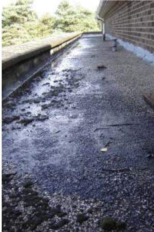
Flat roofs on the west side of the building.
