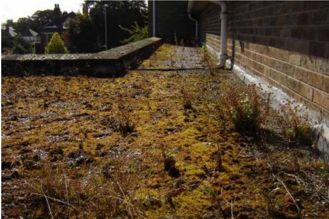
Flat roofs on the east side of the building. An on-going maintenance programme will be required.
