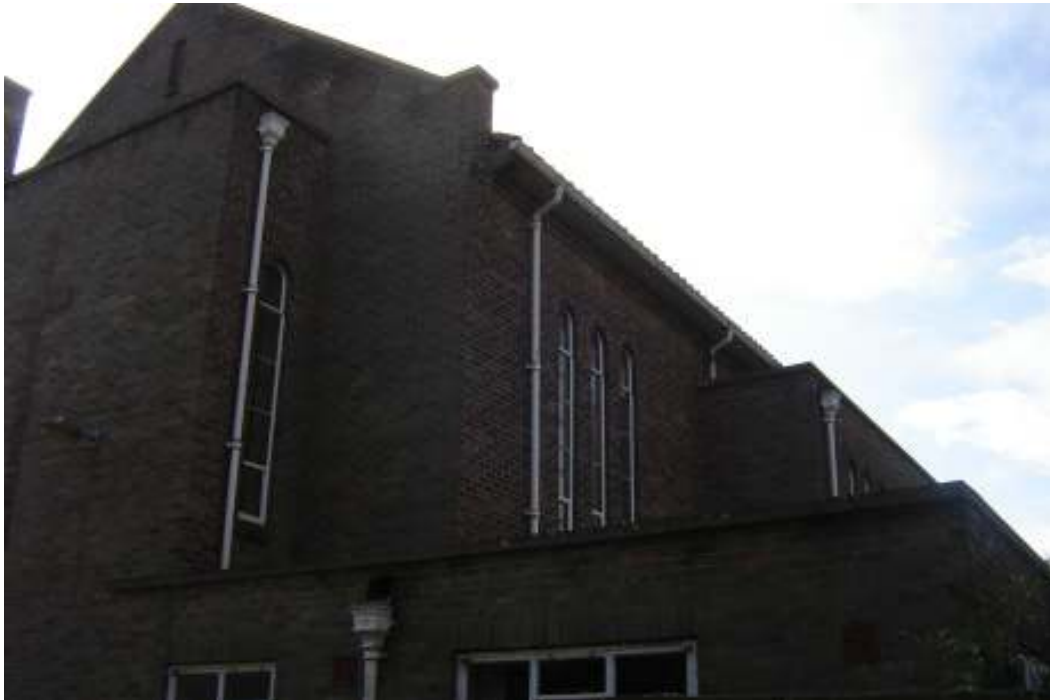
Areas of flat roof north west corner.
